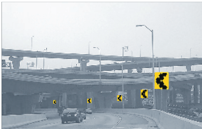
TAPCO's BlinkerChevron™ Dynamic Curve Warning System safely guides drivers through Milwaukee's Marquette Interchange.
